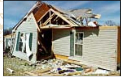
Tornado damage to a house in Georgia, March 20, 1998. See satellite image, next page. Photo by Bill Reckert, Federal Emergency Management Agency (FEMA).
