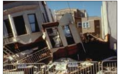
Earthquake damage, San Francisco, October 1989. (NESDIS photo archive.)
