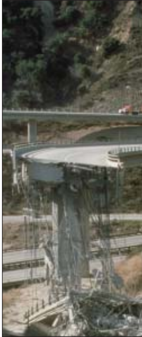
Collapse of the I-5 and SR-14 interchange, Northridge, California, earthquake of 1994. (NESDIS photo archive.)
